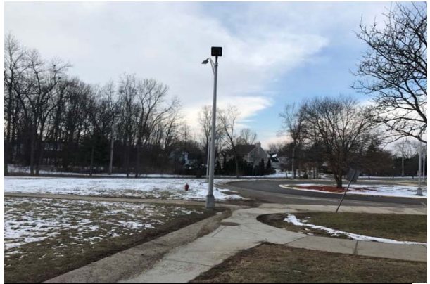
#62: EXTERIOR POLE LIGHT
