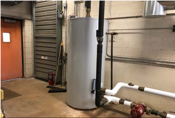
#25: WATER STORAGE TANK
