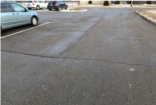
#57: PARKING LOTS, ASPHALT PAVEMENT
