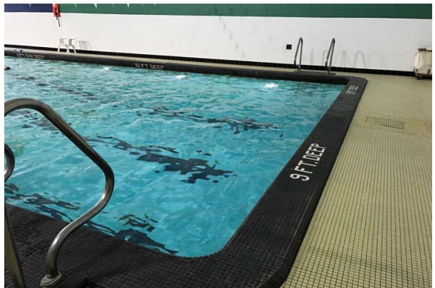
#60: SWIMMING POOL PLASTER
