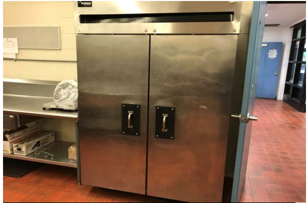
#56: COMMERCIAL KITCHEN, REFRIGERATOR
