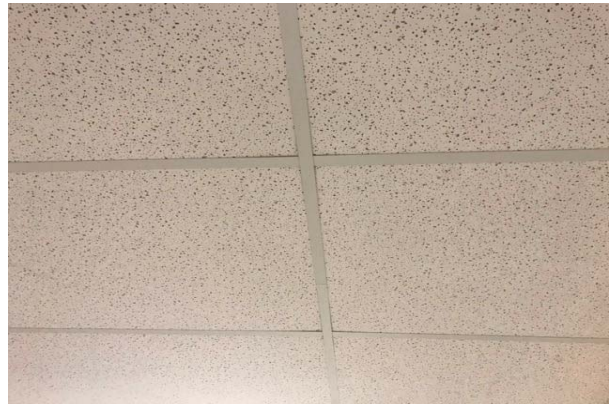
#16: INTERIOR CEILING FINISH, SUSPENDED ACOUSTICAL TILE (ACT)
