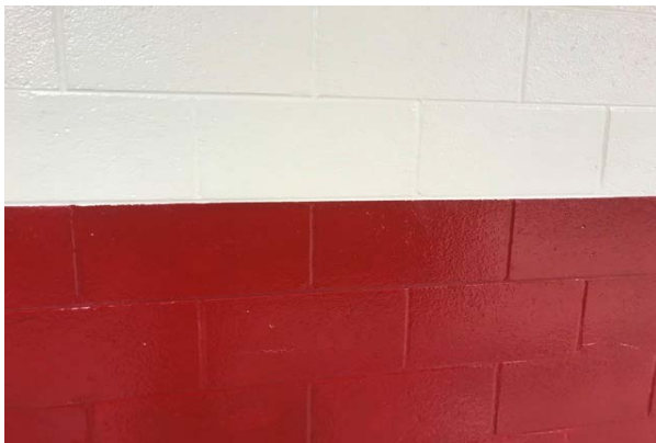
#17: INTERIOR WALL FINISH, CMU
