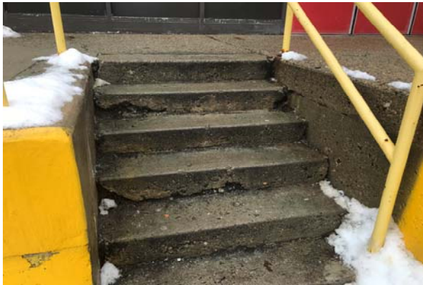
#63: LOADING DOCK STAIRS
