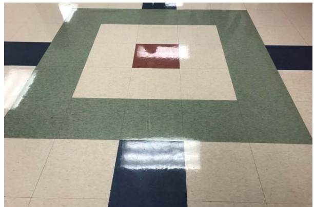
#18: INTERIOR FLOOR FINISH, VINYL TILE (VCT)
