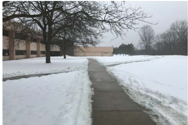
#64: SIDEWALKS AND LANDSCAPING AT REAR ELEVATION
