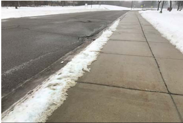
#61: SIDEWALK AND DRIVE AISLE
