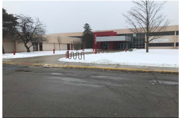
#2: MAIN BUILDING ENTRANCE
