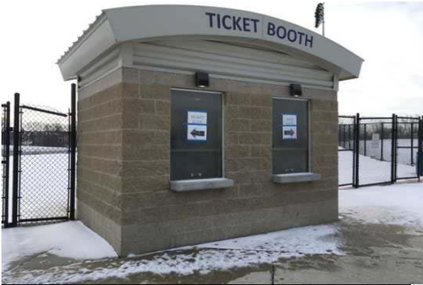
#19: MAIN STADIUM TICKET BOOTH
