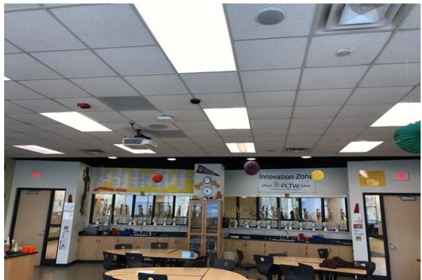
#66: SUSPENDED ACOUSTICAL TILE (ACT) CEILING
